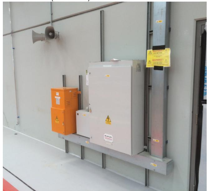
MCB Board (A7183242) and 10 kVA Transformer Distribution Cubicle (A7034165) both with DC Immune RCDs
