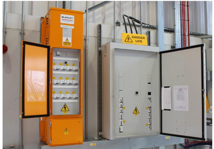
MCB Board (A7183237) and 10 kVA Transformer Distribution Cubicle (A7034241) both with DC Immune RCDs
