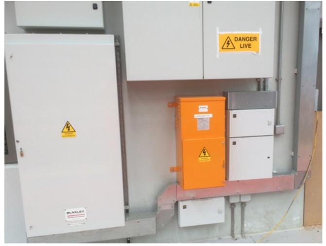
MCB Board (A7183240) and 10 kVA Transformer Distribution Cubicle (A7034163) both with DC Immune RCDs
