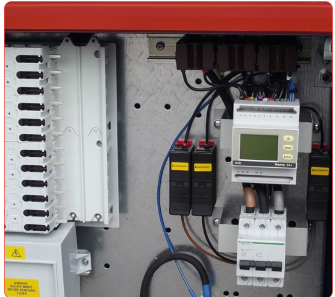
kWhr kit fitted into a B2 series 100A MDA
